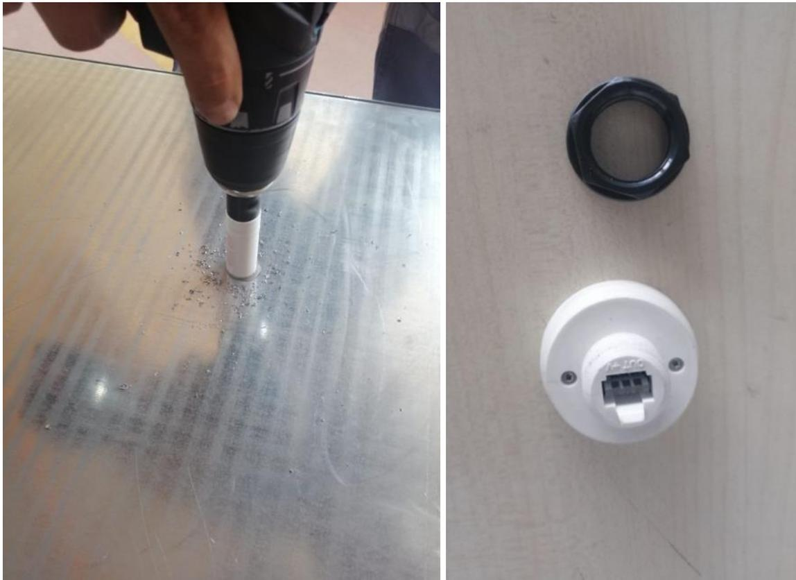
Pass pellet sensor through the 20 mm diameter hole, and secure it with its nut supplied within the package. Having installed, the face with terminal should face the outside of the fuel tank. See following pictures.
