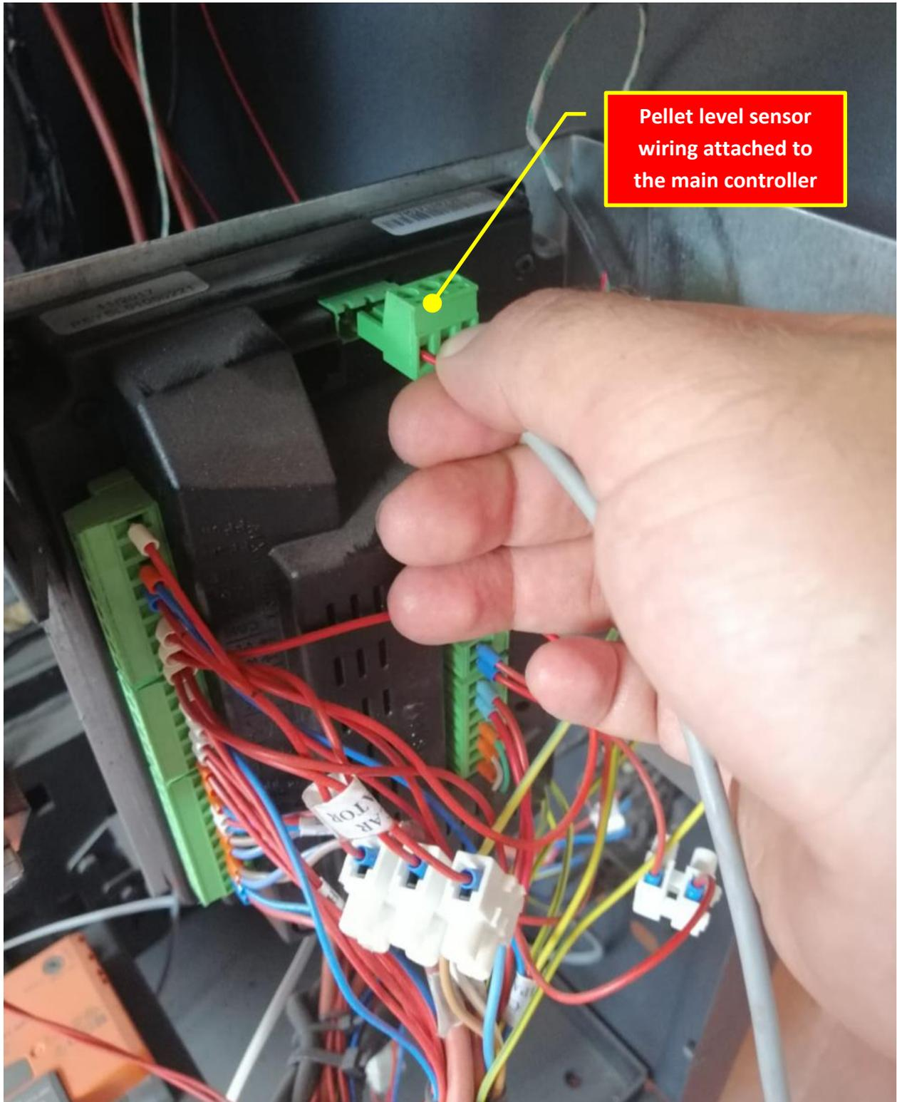
Pellet level sensor wiring attached to the main controller
